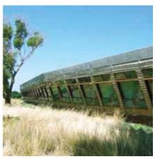
The Outward sloping windows maximise lighting and act as solar controllers. The exposed rough sawn timber imitates coastal architecture where the building faces Swan Bay.
