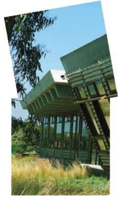
The concrete structure is exposed on the inside and timber cladding insulates from the outside, maximising the benefits of thermal mass.
