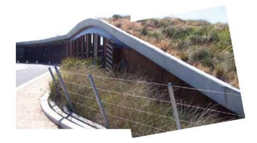
The formal entry to the building (which faces the road) uses more refined timber cladding.
